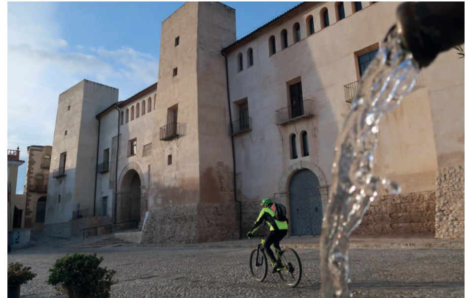
Fortified palace of the Milà and Aragó, Albaida.
